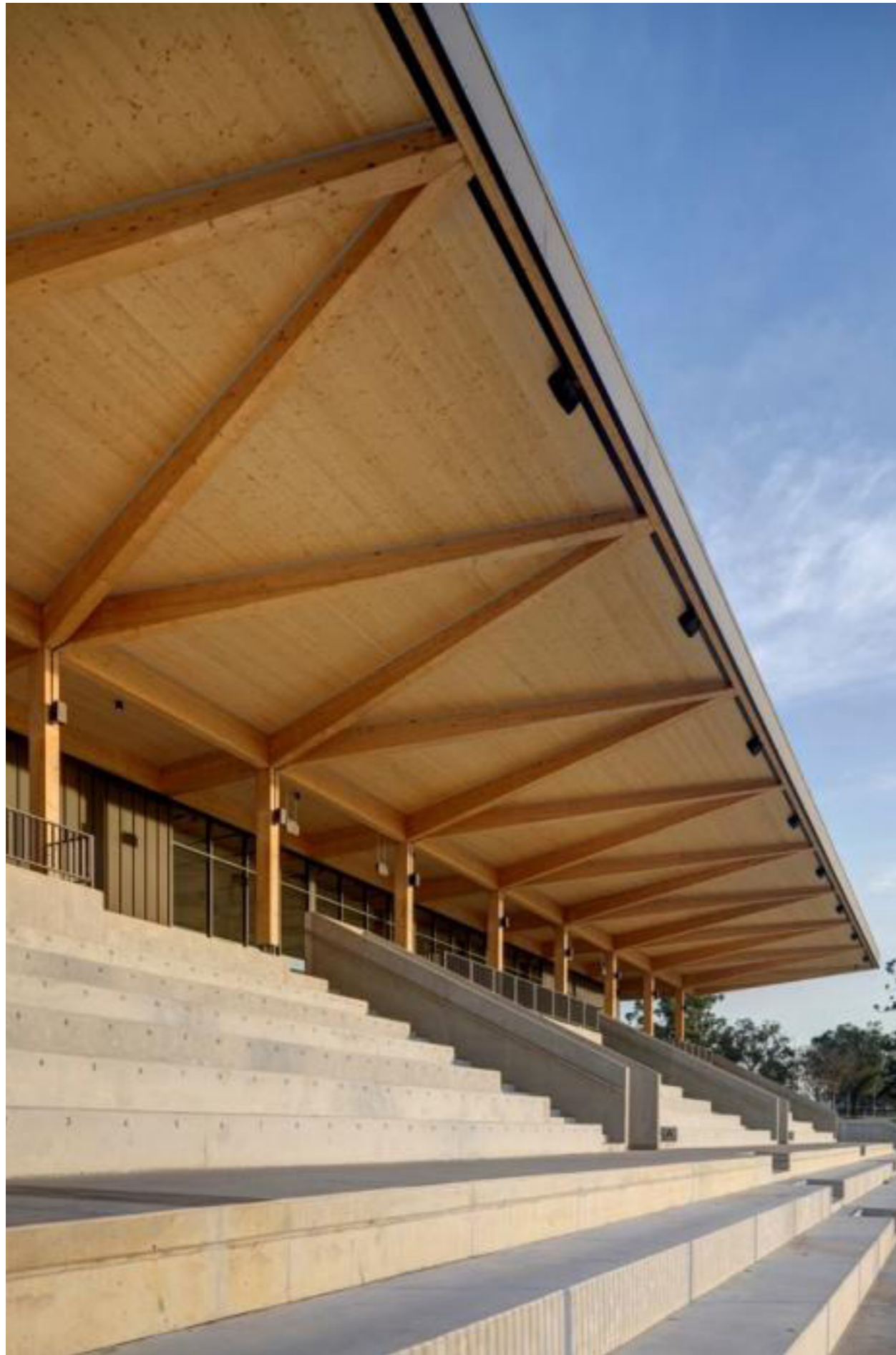
Eric Tweedale Stadium, Sydney, dwp / Northrop, www.northrop.com.au
